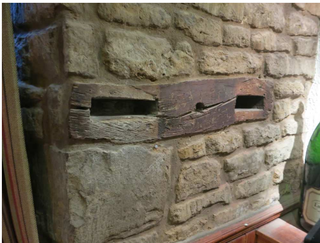
The cruck truss apex, re-set in the wall of west extension
